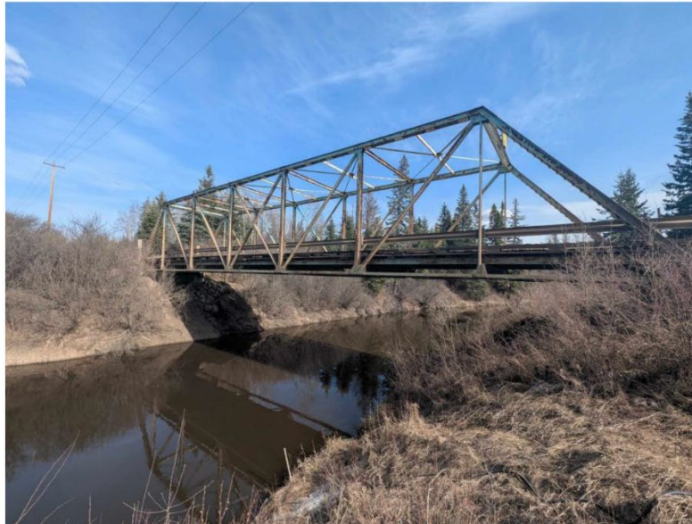
Below: 1931 (placed sometime between 1952-72) steel truss bridge crossing the Redwater River.
