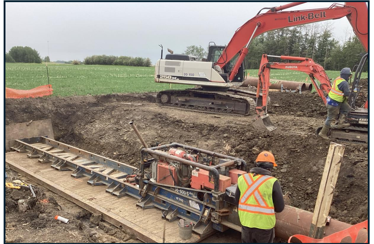
Culvert Coring Twp Rd 554 West of Cardiff
