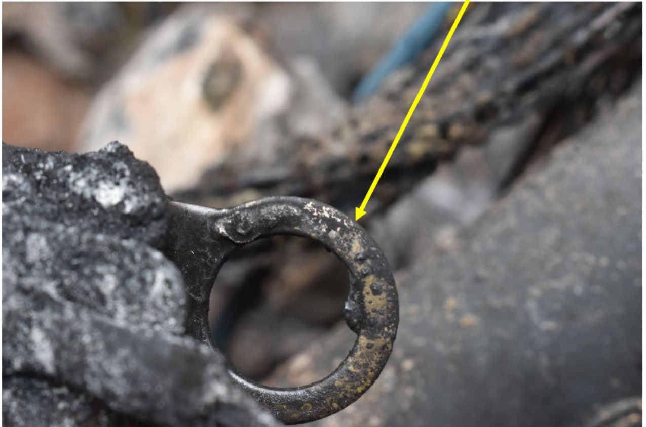
FIGURE 7. FS2025-052 (89), BELOW, CLOSEUP PHOTO OF ARCING ON THE POSITIVE BATTERY CONNECTION.
