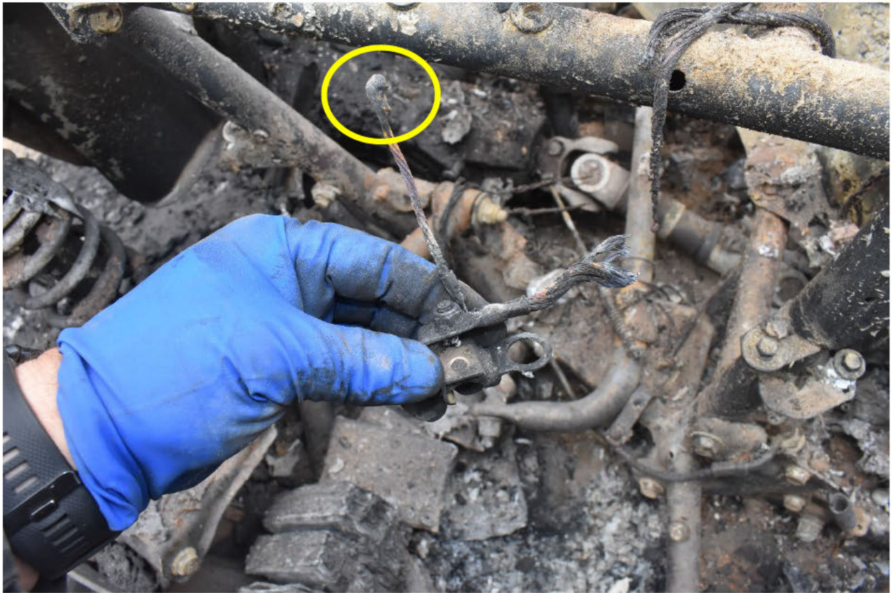
FIGURE 8. FS2025-052 (90), PHOTO OF THE OTHER CONNECTION WIRING FOR THE BATTERY. NOTE THE ARC BEAD.
