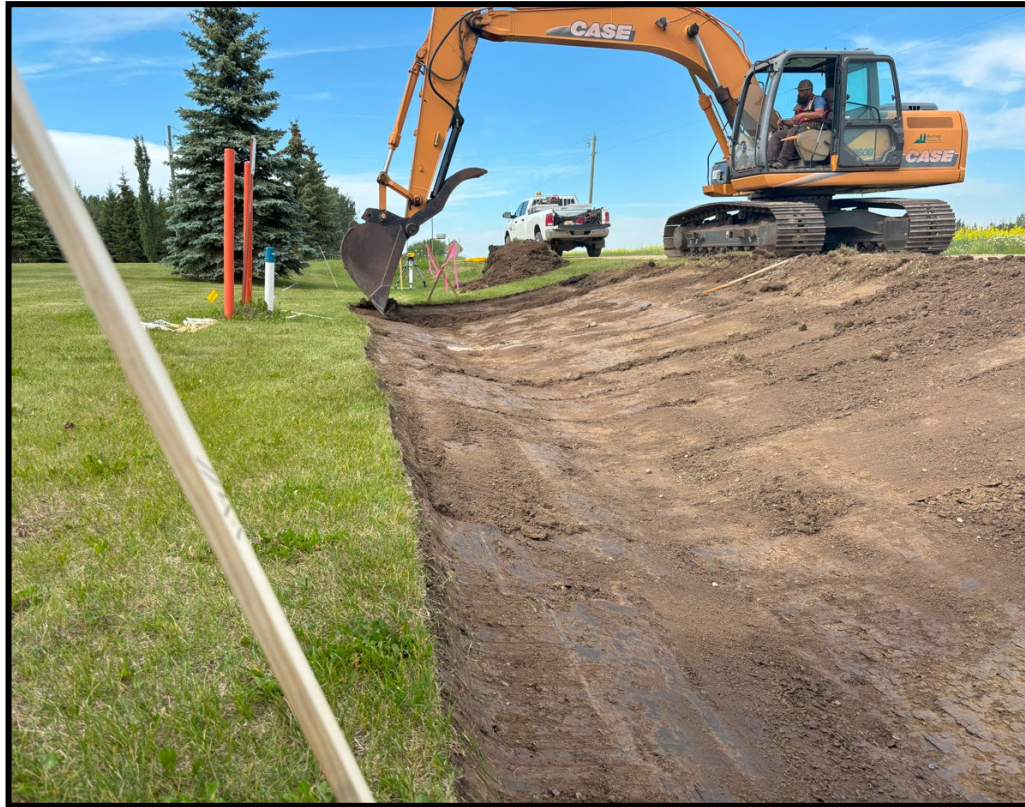
Drainage Improvement Rge Rd 244 South of Twp 564
