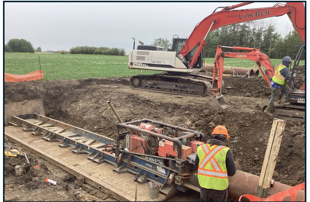
Culvert Coring Twp Rd 554 West of Cardiff
