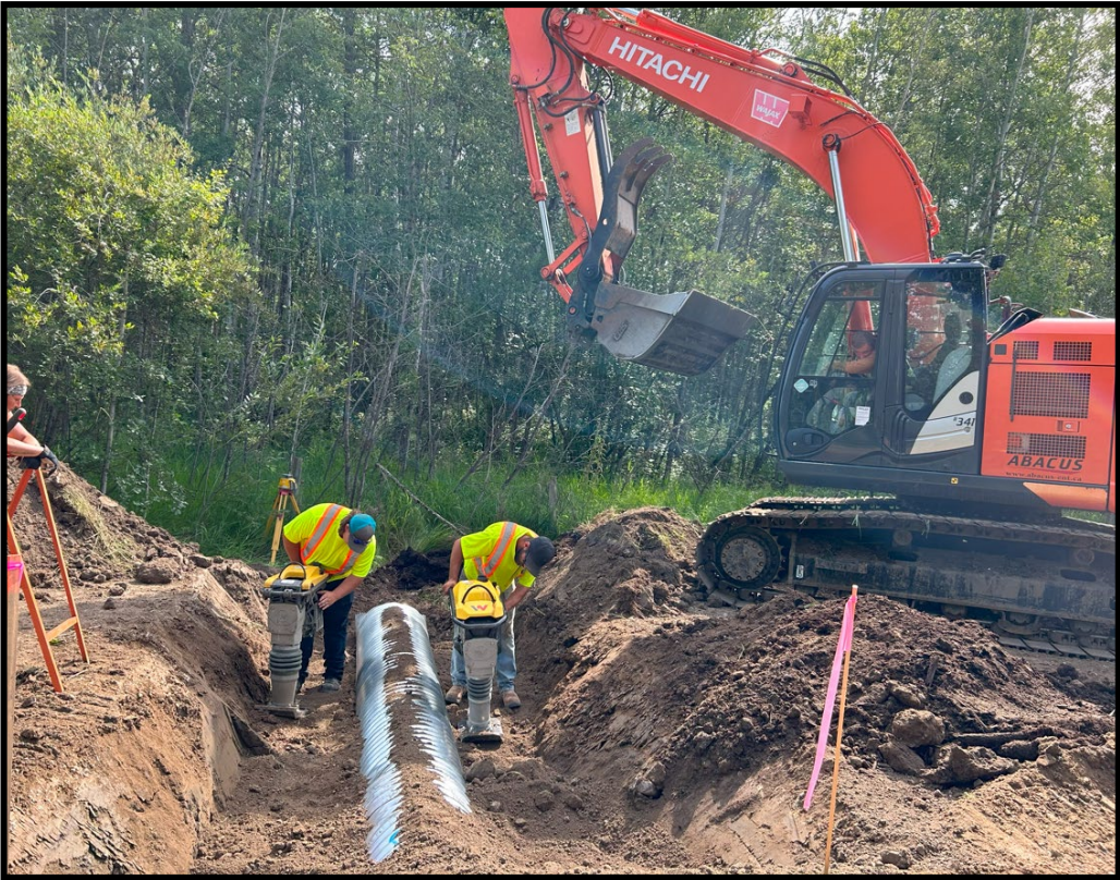
Culvert Replacement Rge Rd 273 North of Twp Rd 540
