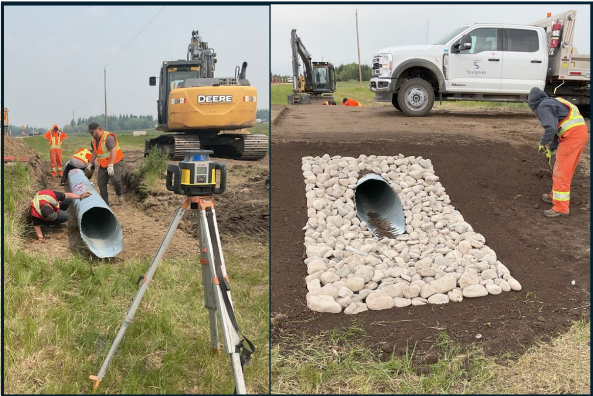
Culvert Replacement Rge Rd 224 North of Hwy 28
