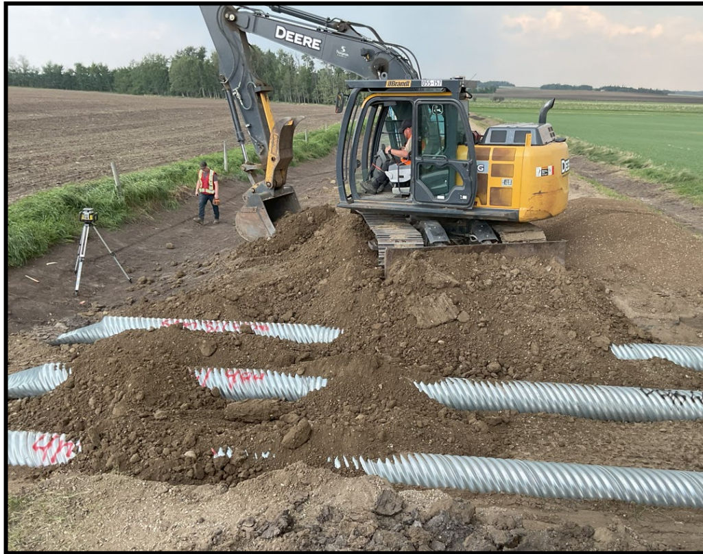
Culvert Replacements and Channel Maintenance Rge Rd 274 North of Twp Rd 564
